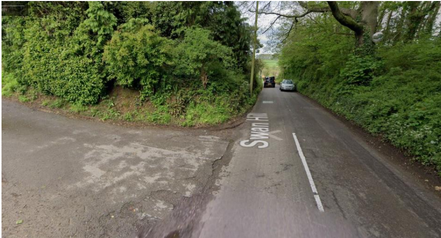
Complete removal of the trees would be needed to give a safe westward vision line
